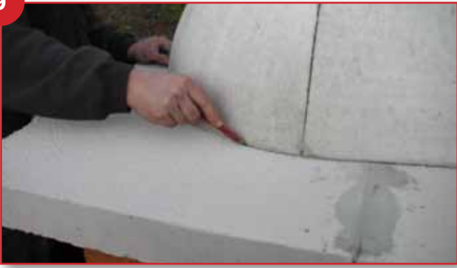
Draw a line around the assembled oven
