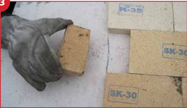
Cut fire bricks to fit making sure the tiles fit up to or just over the drawn line
