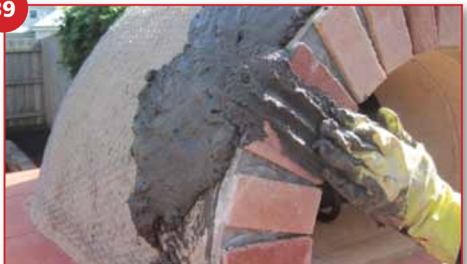
Dampen oven with a fine mist of water (do not saturate) Mix up remaining 3 bags of mortar adding cement colour (not supplied) as required. Start at front of oven working to the back of oven and bringing over the front and into gaps between brick facings
