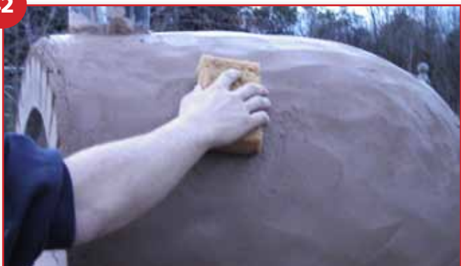
Once you are satisfied with your final shape allow mortar to dry just before mortar sets use a damp sponge in a circular motion to finish off your oven
