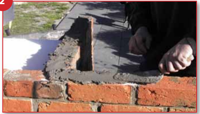
Mix mortar and apply to bricks to secure and level hebel
