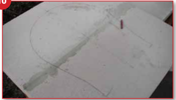
Remove oven shells to expose the drawn line
