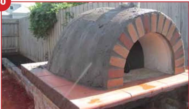
Cover entire oven smoothing by gloved hands applying by rubbing into wire mesh
