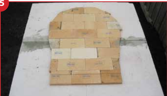
This is how your fire bricks should end up assembled
