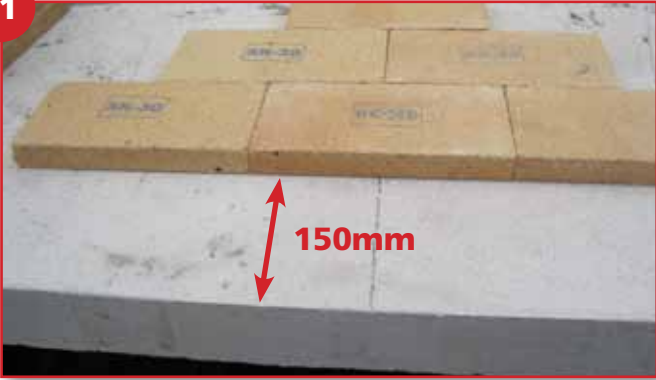
From the front edge of the hebel draw a line at 150mm from edge and align tiles as pictured
