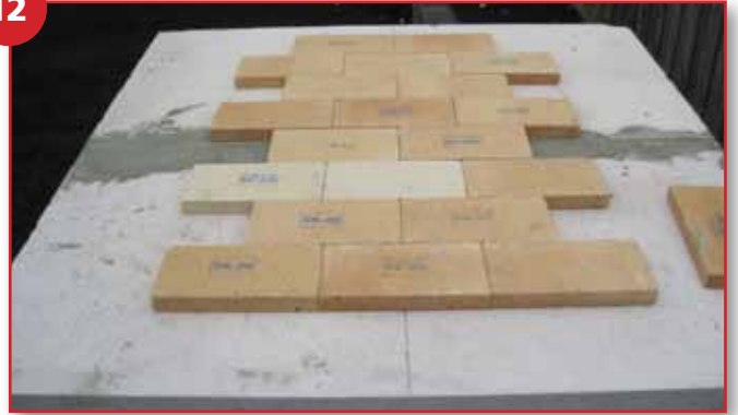
Working toward the back align tiles as pictured
