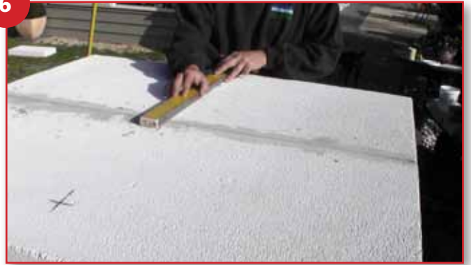
Starting from the front draw a center line on the hebel
