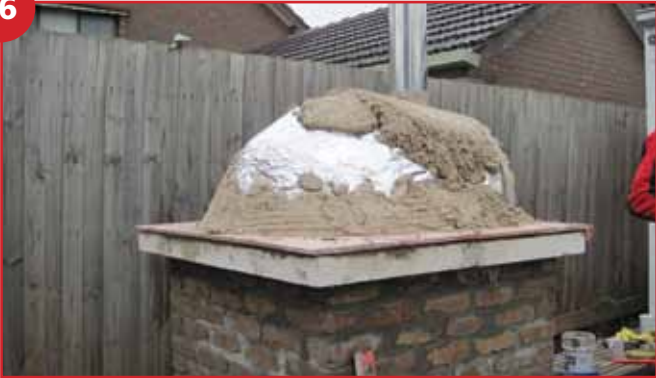
Mix up 4 bags of Shiralite to a paste in a wheelbarrow and working from the front to the back of the oven applying an even depth all over and shaping your oven as you go
