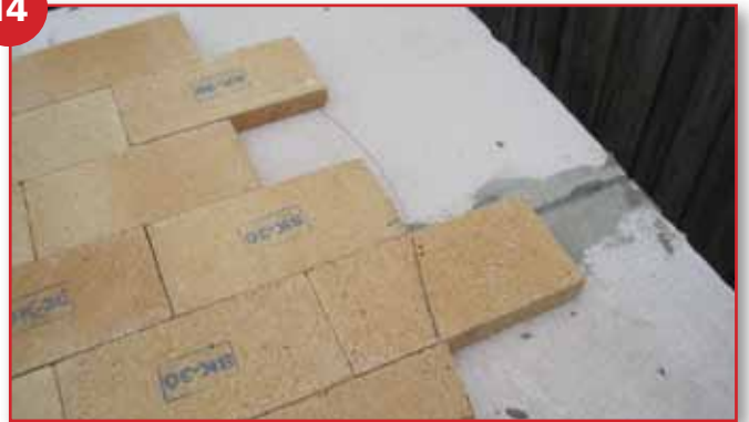
Cut tiles and use off cuts to fill other areas
