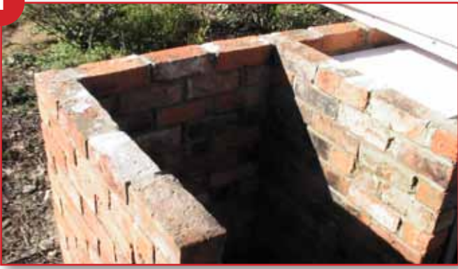
Pictured: Brick Base 1 metre square x 1100 min. height
