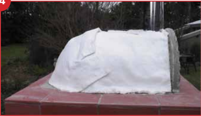
Cover oven with blanket cutting darts to help it shape around the curved areas. Use a mask when handling the blanket material, DO NOT inhale fibres
