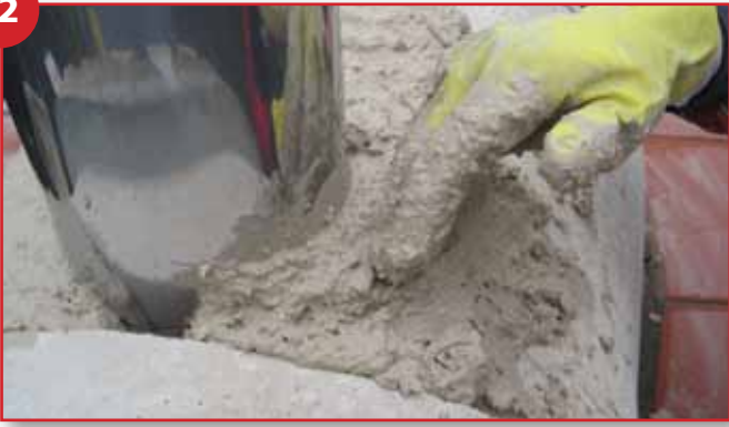
Place Shiracast around the flue as pictured
