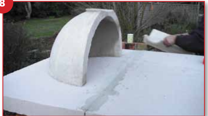
Install the two back half sections of the shells on the hebel starting from the 120mm cross line then install the next two side sections making sure the oven sits square on the hebel
